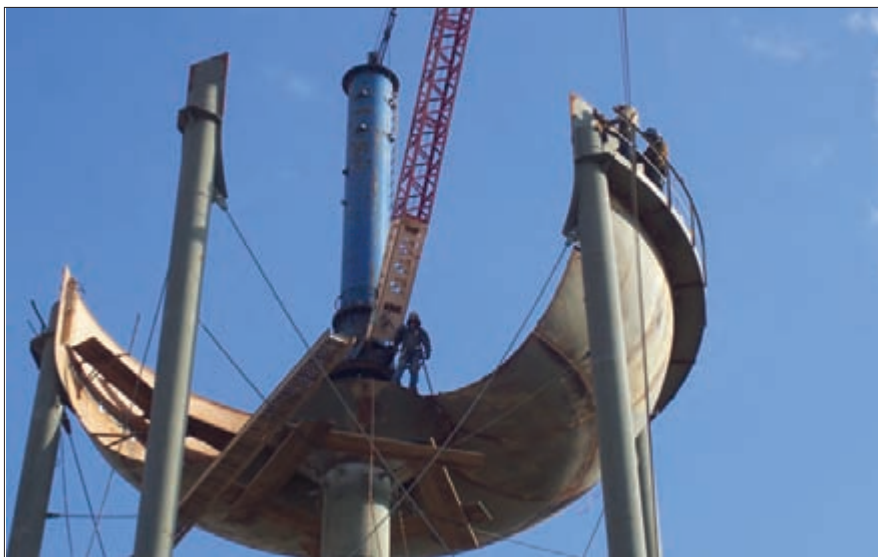
Workers assemble the 250,000-gallon elevated bowl; the tank is 100 feet tall.
