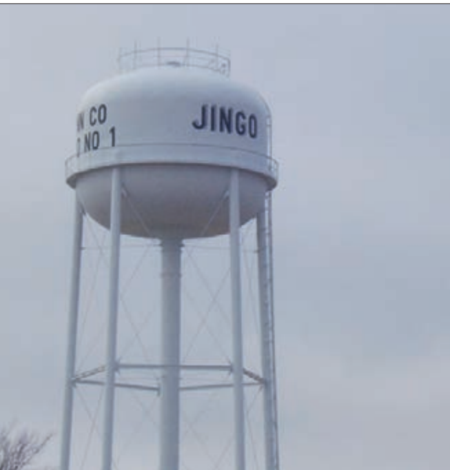
The name JINGO is painted on one side of the storage tank. Doing so was a request of the landowner in memory of the small community in the area.
