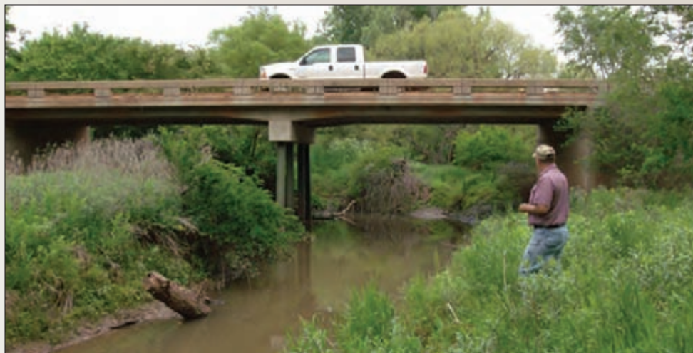
Harper County RWD 4 Operator Jim Coady surveys the location where a 30-gpm leak was located on this crossing. Replacement will involve a directional bore of approximately 250 feet.
