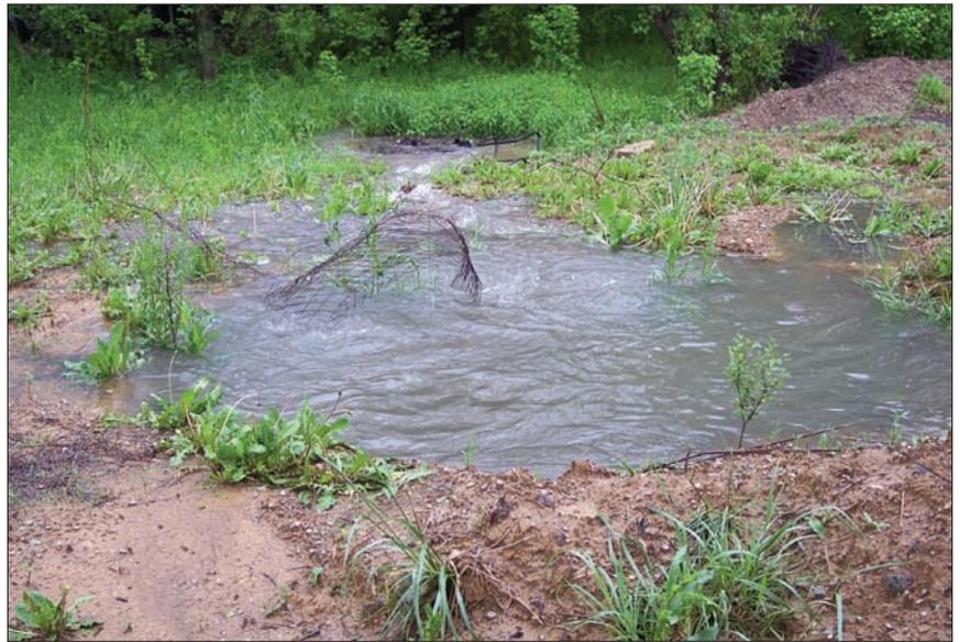
**Believe it or not, there is a manhole located under all that sewage! Due to excessive infiltration and inflow, raw sewage is bypassing from the manhole. Utilities should use their SUO to prohibit illegal connections such as roof drains and sump pumps that can hydraulically overload collection and treatment systems.**
