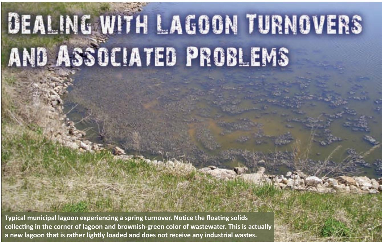
Typical municipal lagoon experiencing a spring turnover. Notice the floating solids collecting in the corner of lagoon and brownish-green color of wastewater. This is actually a new lagoon that is rather lightly loaded and does not receive any industrial wastes.
