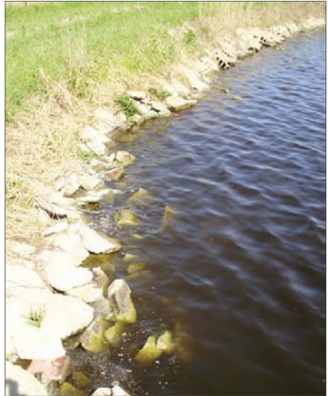
This lagoon cell is experiencing a turnover and lacks the desirable sparkling green color found in a well-operated system. Note the wastewater has a very dark brown color, some white foam developing in the stone rip-rap and very little wave action.
