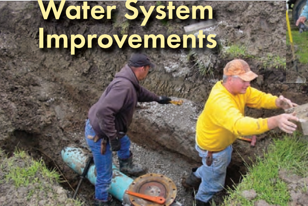
Two crew members of Charlie's Construction, Inc., Frankfort, KS work to install a 10-inch stop in a waterline at Seneca in April 2010. The stop will allow isolation of a section of line to help minimize disruption of service to customers. At right, Charlie Loiseau, owner, Utility Superintendent Brian Rusche, and Seneca Administrator Tami Danliker discuss the work.
