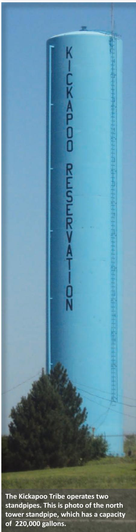
The Kickapoo Tribe operates two standpipes. This is photo of the north tower standpipe, which has a capacity of 220,000 gallons.
