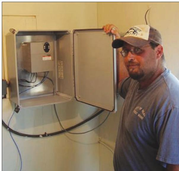
**City Manager Alan Brown is pleased with the operation of the new variable frequency drives installed recently to help control well pumps.**
