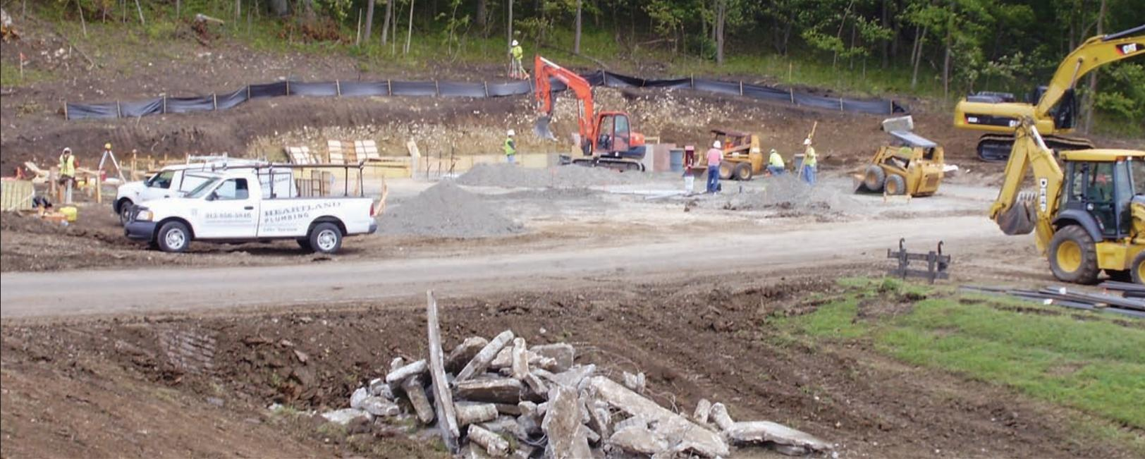
**Grimm Construction employees prepare the foundation for new headworks building that will house mechanical bar screens and grit removal facility.**
