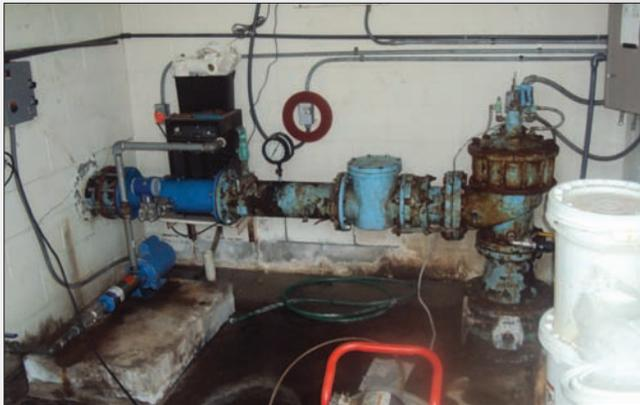
**Before:** This photo shows a pump station as found by KRWA staff in a northeastern Kansas rural water district: plugged drain, cracked wall, rusting equipment and piping. The operator abruptly resigned.
