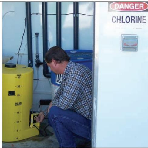
**Tony Kimmi adjusts chlorine feed rate in one of the rechlorination stations provided as a service to water systems in critical need of rechlorination. KRWA has constructed several of such stations.**
