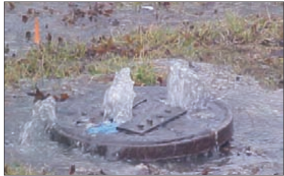
This photo vividly demonstrates the effects of excessive inflow and infiltration during a heavy rain event.
