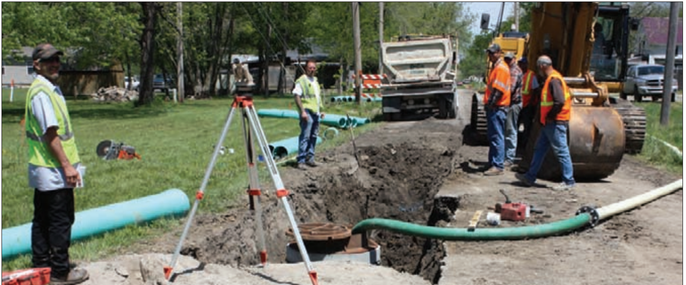
EmCon, Inc. was the contractor on the Burlingame project.
