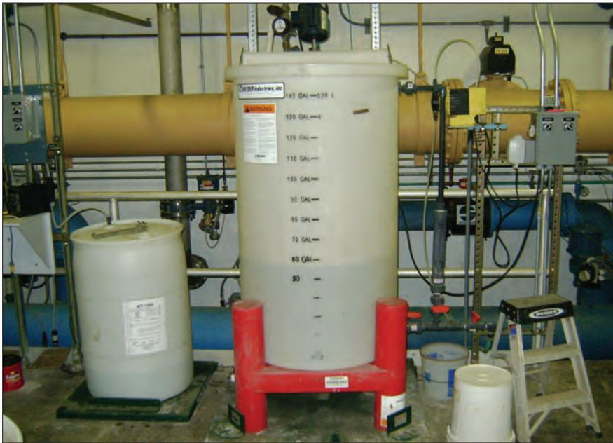
Daily usage for calculating ammonia dosage is measured by graduations on the tank to show how much ammonium sulfate solution is used.
