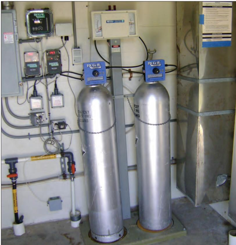
Daily gas chlorine usage in pounds is measured with weight scales. Then the pounds used can be used to calculate the free chlorine dosage.
