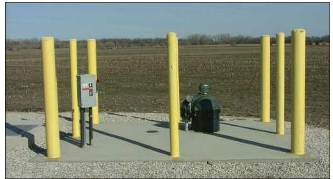
This photo shows the new well located seven miles south of Hoisington. The wellhead was elevated for protection from surface water and further protected with concrete slab and guard posts.
