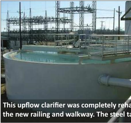
This upflow clarifier was completely rehabilitated with new interior equipment. Notice the new railing and walkway. The steel tank is the original tank installed in about 1960.
