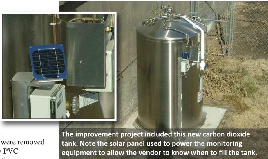
The improvement project included this new carbon dioxide tank. Note the solar panel used to power the monitoring equipment to allow the vendor to know when to fill the tank.
