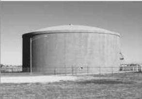
**Prestressed Concrete Water Storage Tanks**
