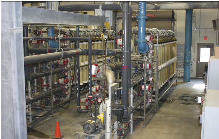
PWWSD 18's original membrane filter system was installed in a new plant in 2002. By late Spring 2013, the district will switch from the membranes to conventional rapid sand filtration.
