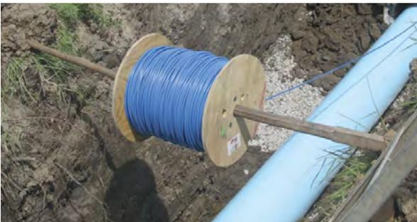
PVC pipe is being pulled through along with tracer wire.
