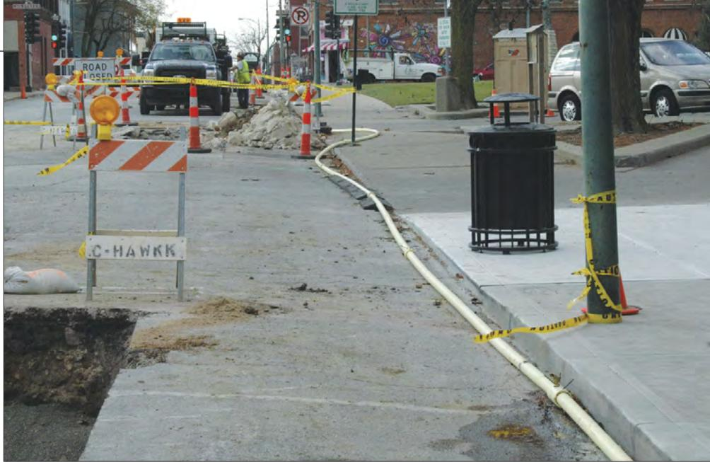
Two cuts were made on the downtown project on Shawnee Street with undisturbed street between the cuts. Note the 2-inch yellow mine pipe used to continue service to customers during the main line replacement procedure.
