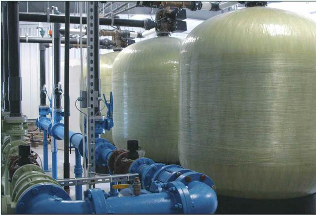
The nitrate removal plant for the city of Woodston includes these three fiberglass exchange vessels and related piping. The tanks contain nitrate selective resin provided by Krudico, Inc. The regeneration process consists of backwash at 40 gpm for 10 minutes, brine draw slow rinse at 20 gpm for 25 minutes, slow rinse at 10 gpm for 35 minutes, and fast rinse at 40 gpm for 12 minutes.
