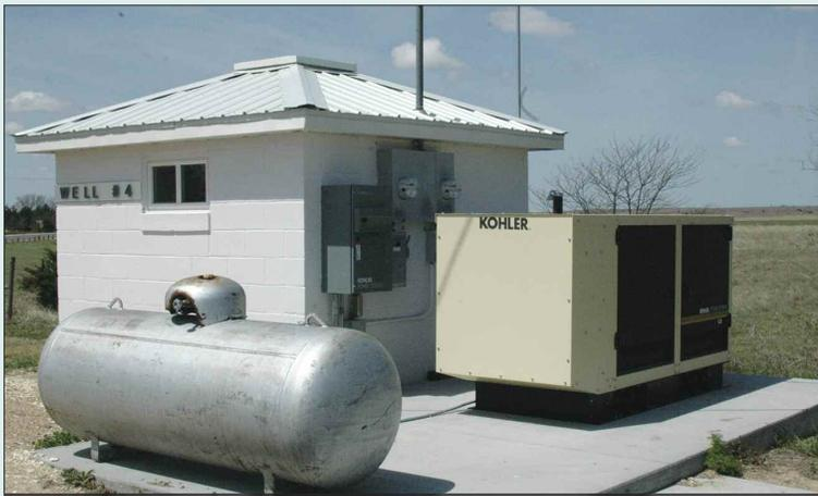
Well No. 4 was rehabilitated with new piping and a new 15 HP pump and motor. A standby generator was also provided at this well.
