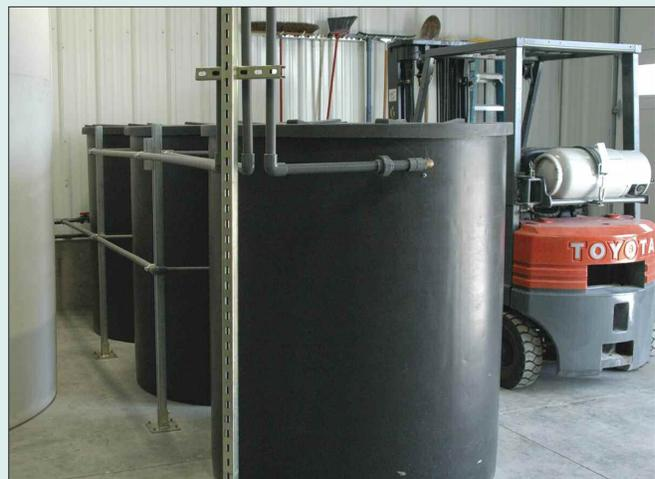
This photo shows the relative location of the black tanks with salt brine solution used to regenerate the resin in the exchange tanks, waste water storage tank, and the forklift used for handling pellets of salt bags.
