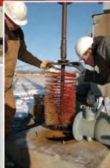
In a well remediation, Alexander Pump's unique truck mounted hydraulic walking beam (above) cycles the surge tank, double surge block and brush (left) up and down through the well. The action forces 'Redi Clean' chemicals into the gravel pack to dissolve iron bacteria, placing it into suspension for removal.
