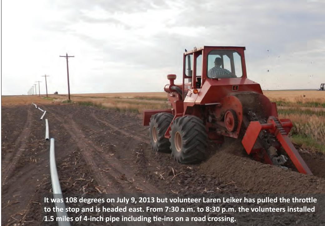
It was 108 degrees on July 9, 2013 but volunteer Laren Leiker has pulled the throttle to the stop and is headed east. From 7:30 a.m. to 8:30 p.m. the volunteers installed 1.5 miles of 4-inch pipe including tie-ins on a road crossing.
