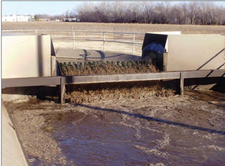
**Close-up of operating rotor which provides DO needed for aerobic zone directly downstream. The rotor rpm varies based on set-point selected by the operator. The rotor also provides mixing and ensures solids remain suspended in mixed liquor.**
