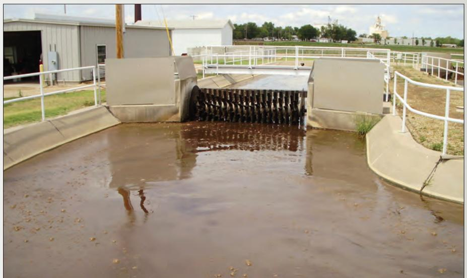
**This "off-rotor" is operated at very low rpm so that oxygen is not increased in anoxic zone, but mixed liquor solids stay suspended.**
