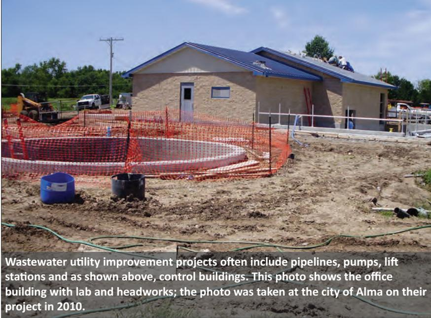
Wastewater utility improvement projects often include pipelines, pumps, lift stations and as shown above, control buildings. This photo shows the office building with lab and headworks; the photo was taken at the city of Alma on their project in 2010.
