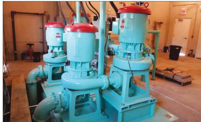
**Influent pump station must pump against a 200-foot head to the lagoon almost four miles from town. The Smith & Loveless 75 hp pumps are paired together and pump in series. Each pair of pumps can pump 750 gpm.**
