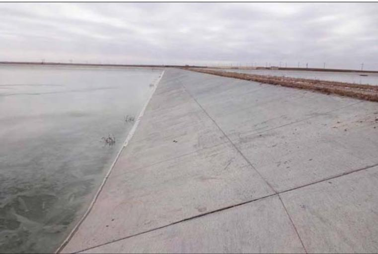
All three lagoon cells have concrete aprons such as this to prevent erosion problems. This is especially critical on Cell 3 where the water depth can vary from five feet to nine feet.
