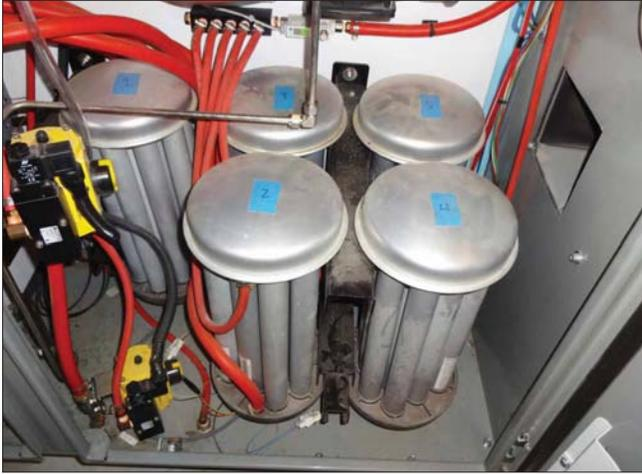
**These scrubbers are used to separate nitrogen so that high-purity oxygen remains. Some of the oxygen is then used to produce ozone on-site. Ozone and oxygen are usually fed together as each creates specific benefits. Ozone is effective at controlling sulfate-reducing bacteria that cause odors. Oxygen ensures anaerobic conditions do not develop.**
