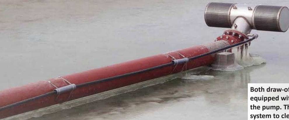
Both draw-off pipes to the Effluent Pumping Station are equipped with screens to prevent solids from damaging the pump. The station is also equipped with an air purge system to clear the screens before pumping begins.
