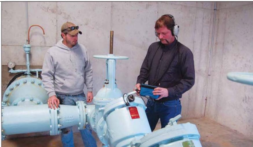
**Josh Van Tyal, Operator for Suburban Water Company, watches as Tony Kimmi listens to the dual 12-inch check valve for possible backflow. This installation is at interconnection between Suburban Water and BPU, Kansas City.**
