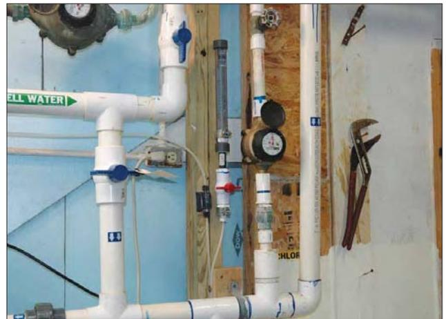
**This new meter was installed in the bypass line to allow raw well water to blend with softened water. The goal is to produce water to customers that will be lower in sodium and not as aggressive to metal piping as water with very low Total Hardness.**
