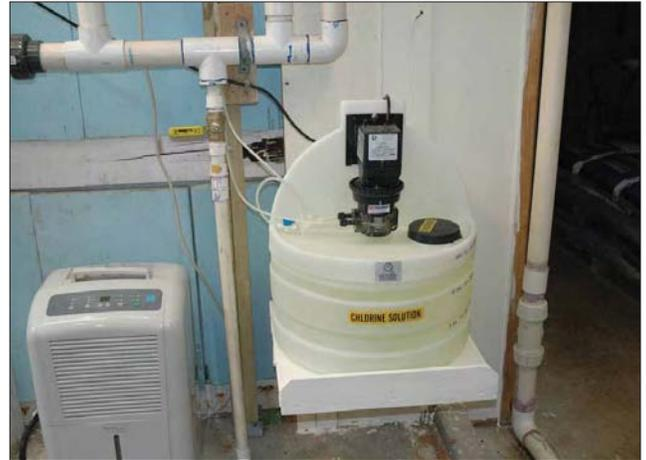
**This new solution tank and a peristaltic pump were installed by KRWA Tech Assistants Lonnie Boller and Tony Kimmi. This equipment is appropriately sized for the low rate of flow through the plant. The city's two wells only produce a total of 22 to 25 gpm.**
