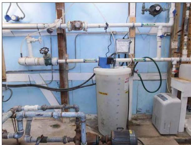
This photo shows the large solution day tank used prior to changing out the chlorination equipment at the city of McFarland, KS. The operator was diluting 10% sodium hypochlorite on a daily basis and at times would find the tank empty when he would return to check the system. The original pump was over-sized for the rate of the water flow through the plant.
