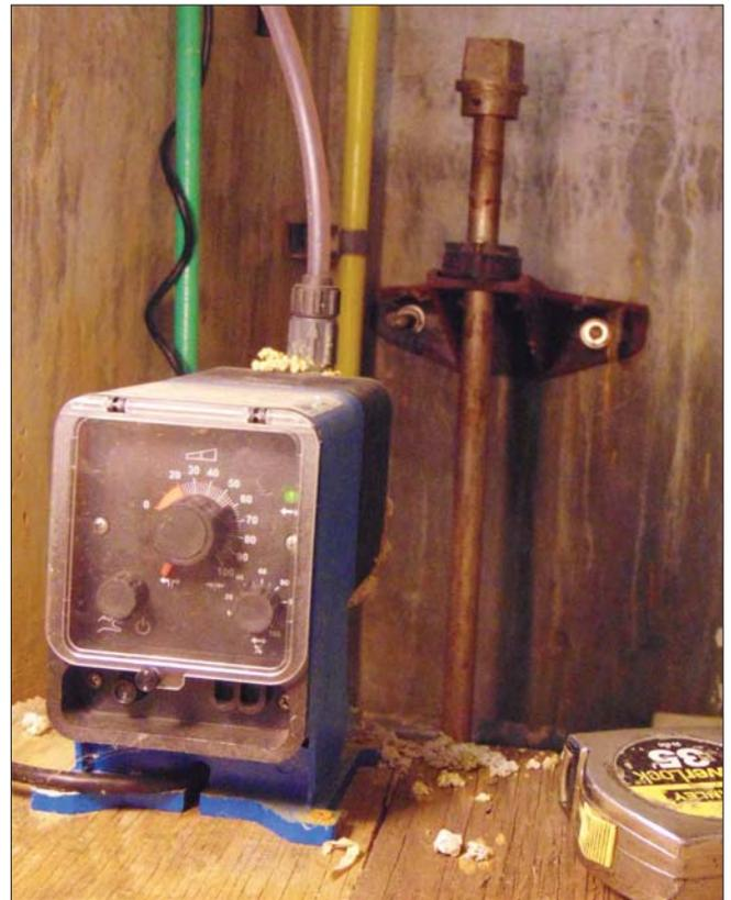
**These chemical feed pumps are used to inject ferric sulfate to reduce total phosphorus.**
