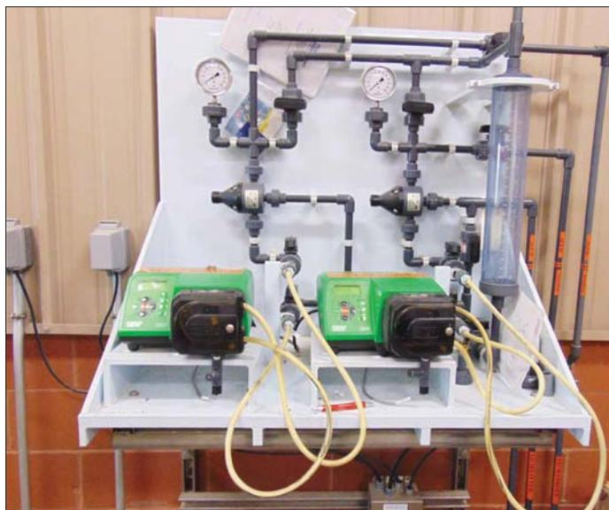
These pumps add the alum to reduce the total phosphorus to meet limits of 0.5 mg/L in a Kansas wastewater system.
