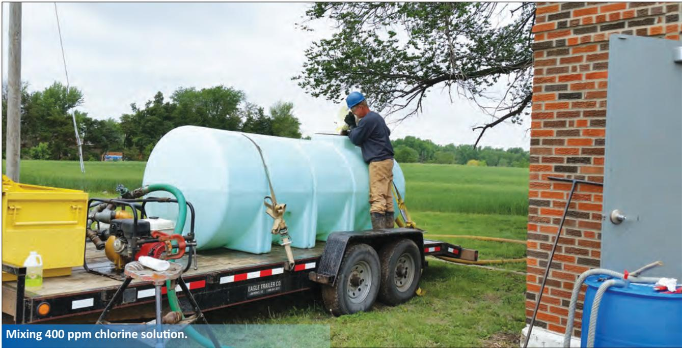
Mixing 400 ppm chlorine solution.
