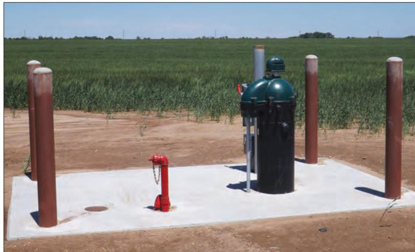
This is one of two new wells providing water for the Sumner RWD 5. Each well will provide 425 gpm to the system.
