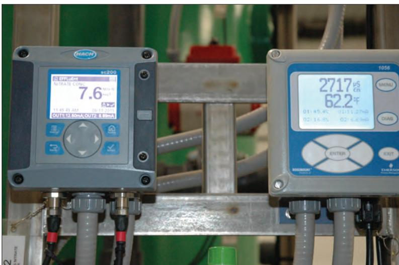
This display shows the level of nitrate (7.6 mg/L) being delivered to customers. The nitrate level can be controlled by the amount of raw well water being blended with treated water.
