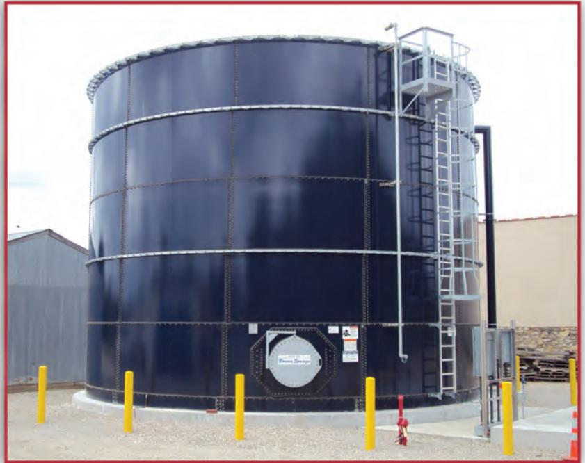
The water system improvements at Bonner Spring, KS include this 130,000-gallon glass-lined settling tank where iron and manganese settles out in the treatment process.
