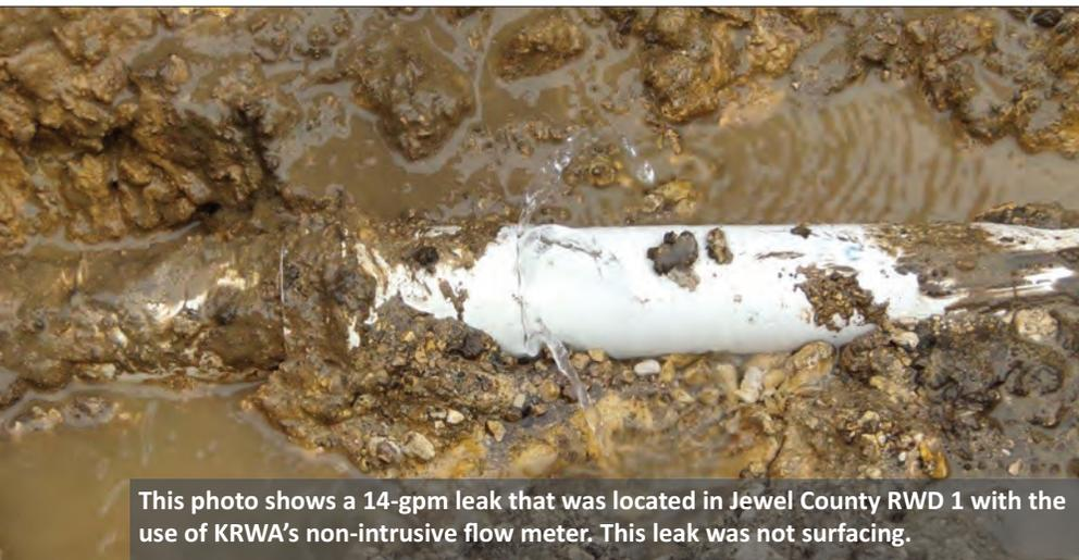
This photo shows a 14-gpm leak that was located in Jewel County RWD 1 with the use of KRWA's non-intrusive flow meter. This leak was not surfacing.
