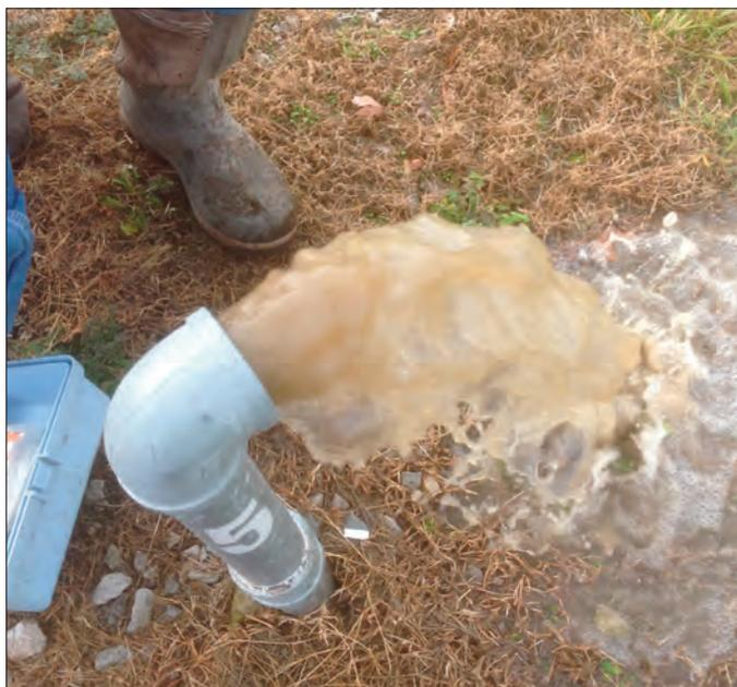
This photo shows discolored water being pumped during extended flushing of Well No. 5 following super-chlorination.
