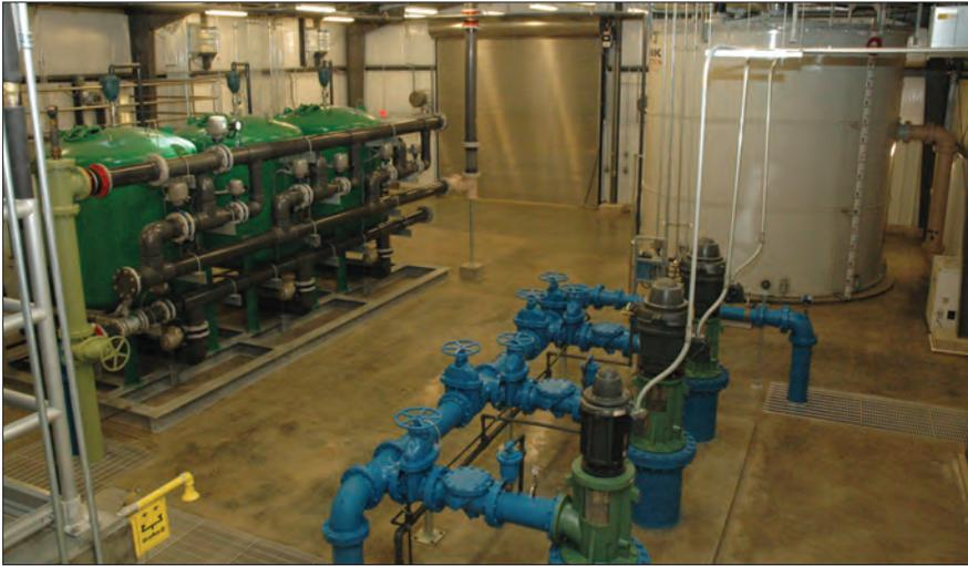
This photo in Smith Center's new treatment plant shows the high service pumps, the LayneOx filters on the left, and the backwash holding tank in the background.
