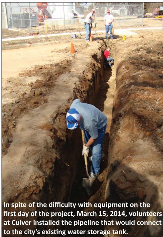
**In spite of the difficulty with equipment on the first day of the project, March 15, 2014, volunteers at Culver installed the pipeline that would connect to the city's existing water storage tank.**
