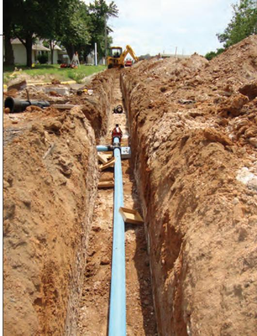
**The water system improvement project in Turon is being funded through a \$300,000 KAN STEP Grant. This photo shows how local people can cut a straight ditch with a backhoe.**
