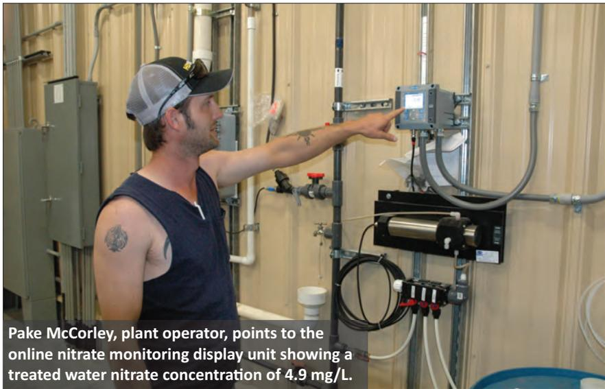
Pake McCorley, plant operator, points to the online nitrate monitoring display unit showing a treated water nitrate concentration of 4.9 mg/L.
