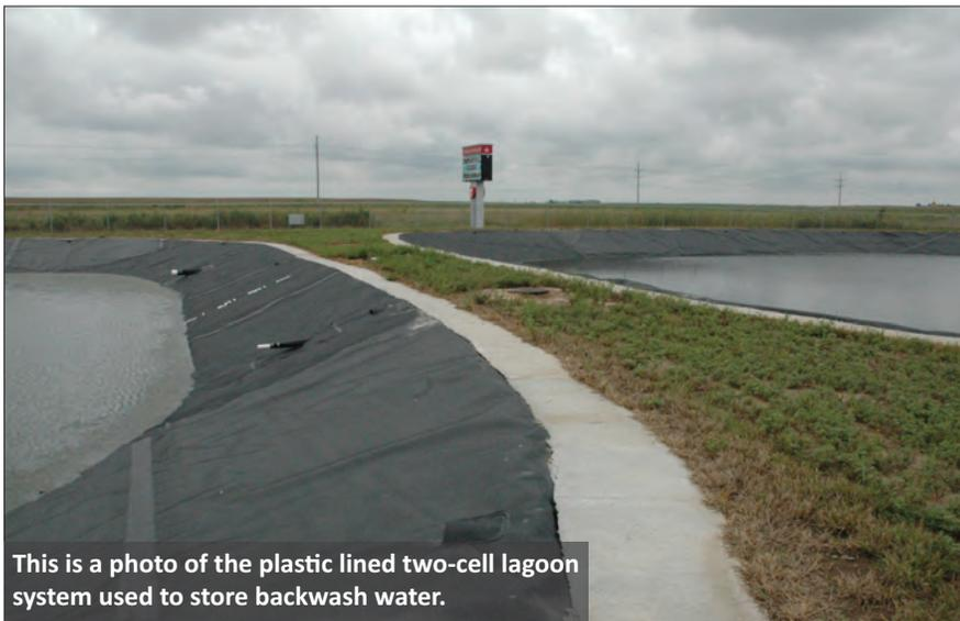
This is a photo of the plastic lined two-cell lagoon system used to store backwash water.
