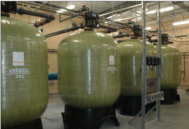
Four ion-exchange tanks are used to remove nitrate.
