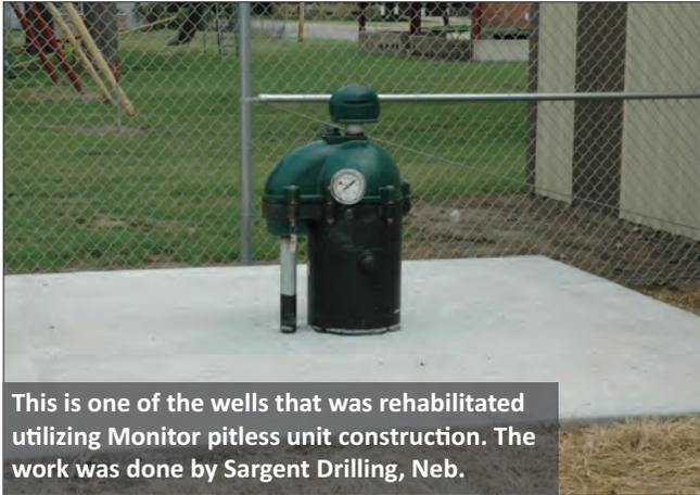
This is one of the wells that was rehabilitated utilizing Monitor pitless unit construction. The work was done by Sargent Drilling, Neb.
