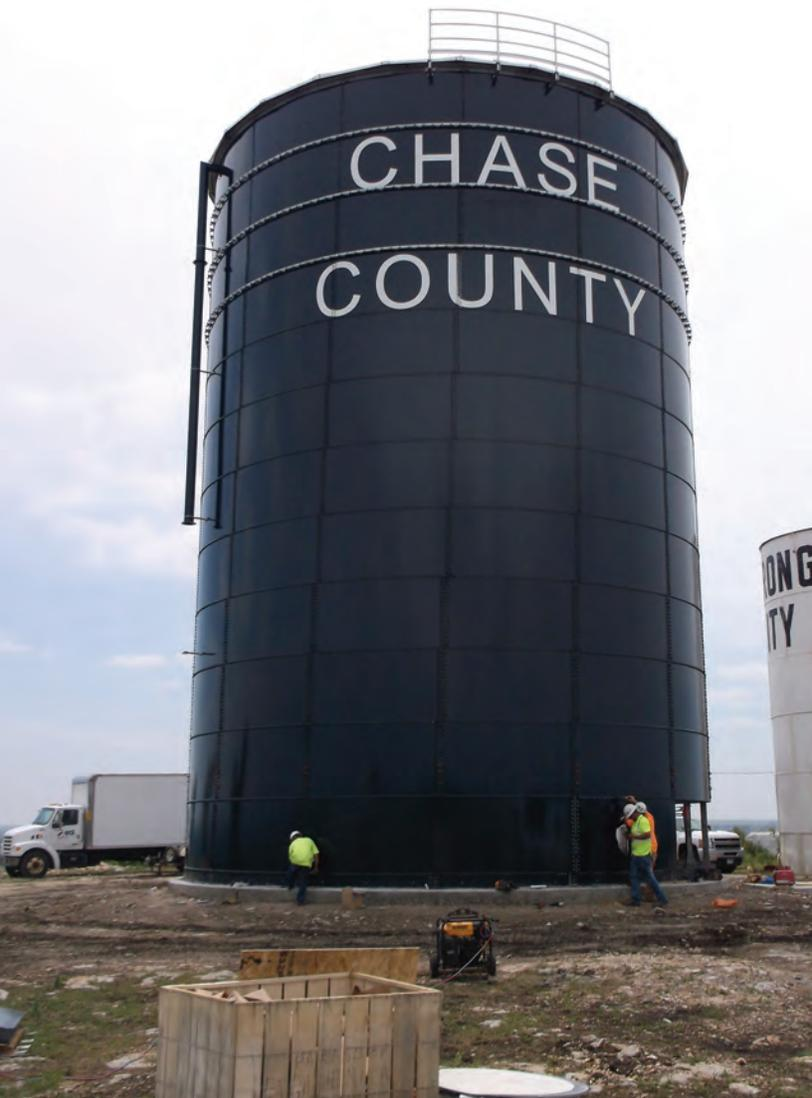
This 0.5 MG water storage tank was constructed next to Strong City's original ground storage tank on a hill east of the city. Under construction in late 2015, this is the only tank that supplies water storage and pressure to the three entities of Public Wholesale District No. 26 – Strong City, Cottonwood Falls and Chase RWD 1.
