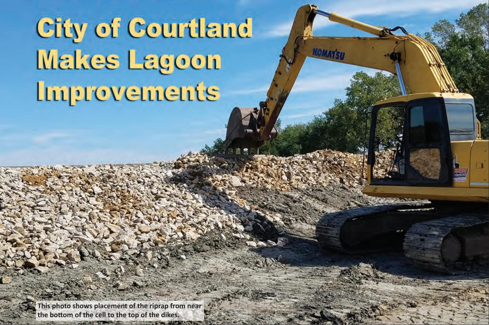
This photo shows placement of the riprap from near the bottom of the cell to the top of the dikes.
