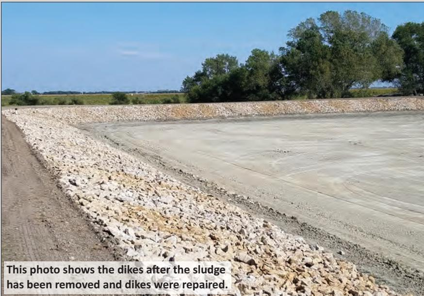
This photo shows the dikes after the sludge has been removed and dikes were repaired.
