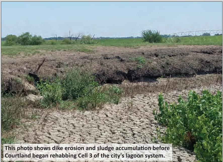
This photo shows dike erosion and sludge accumulation before Courtland began rehabbing Cell 3 of the city's lagoon system.
