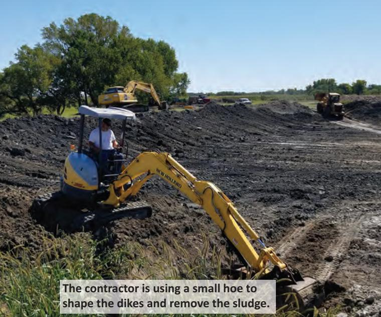
The contractor is using a small hoe to shape the dikes and remove the sludge.
