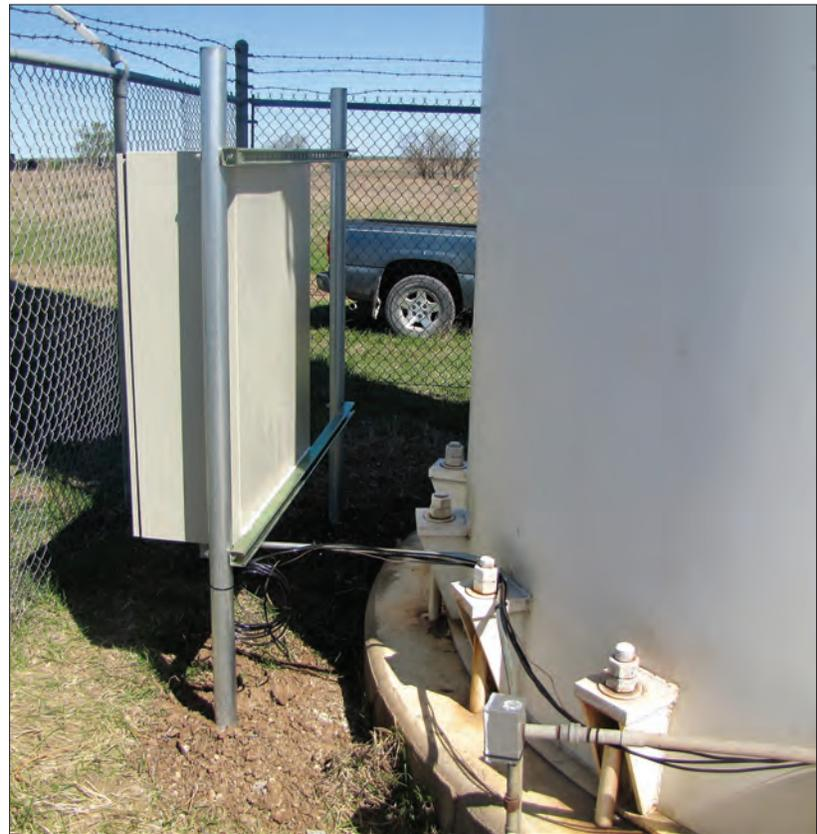
**This photo shows anchor bolts on a water standpipe in Butler RWD 4. Taps had loosened several rounds of threading.**
