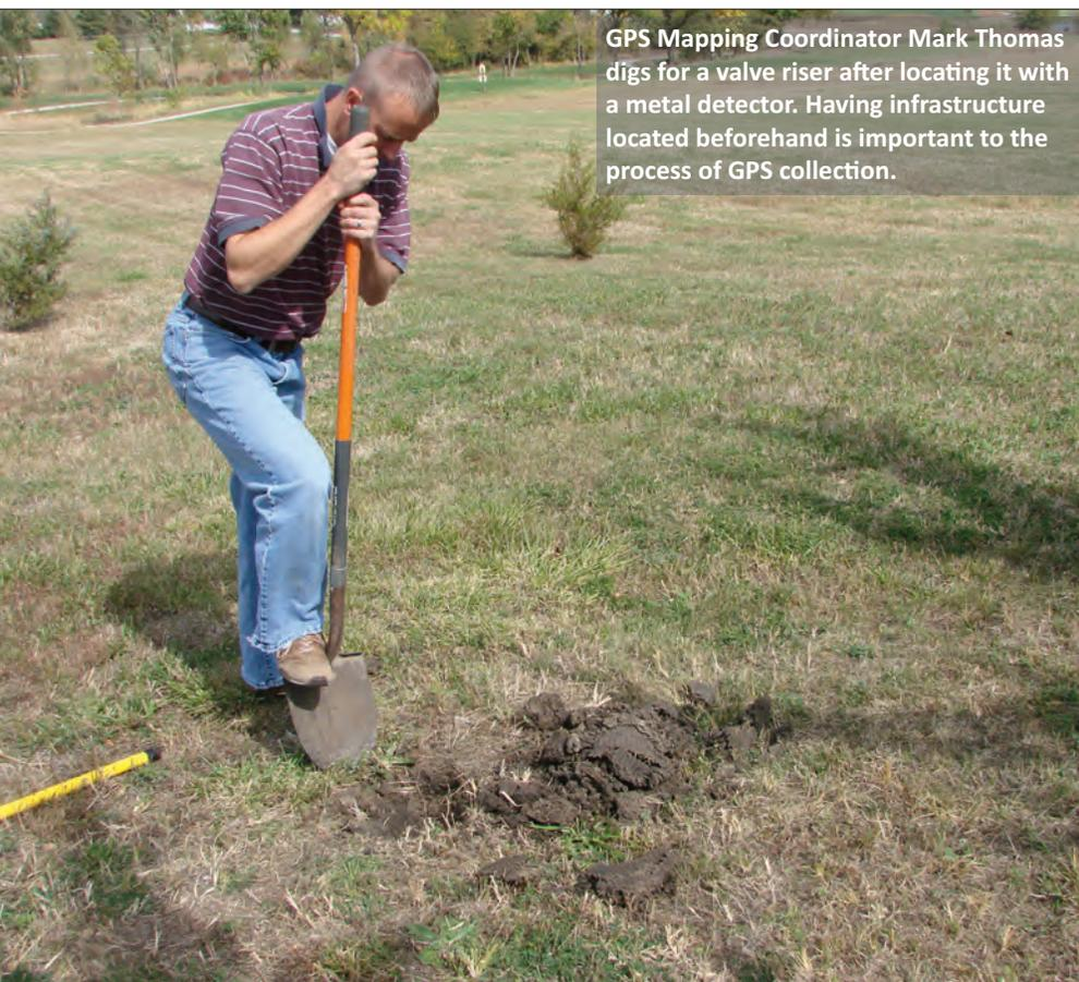
GPS Mapping Coordinator Mark Thomas digs for a valve riser after locating it with a metal detector. Having infrastructure located beforehand is important to the process of GPS collection.
