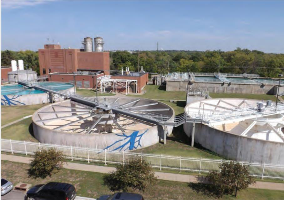
This photo shows three of the basins in the foreground (two not currently in use), the chemical building in the background (left), and the river settling basin in the background right.
