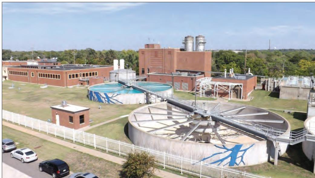
**This overhead view of the 20 MGD water treatment plant treats groundwater from 15 wells and surface water from the Smoky Hill River. Total raw water pumped in 2016 was 2.0 billion gallons, with 1.3 billion gallons (65 percent) from groundwater and 0.7 billion gallons (35 percent) from surface water.**
