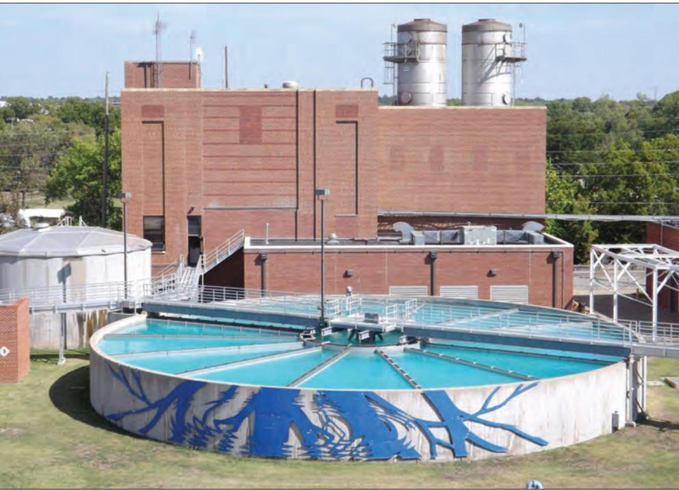
There are a total of four basins at this plant. Two are softening basins and two are secondary settling basins. This photo shows one of the basins in the foreground and the chemical building and the two aeration towers in the background.
