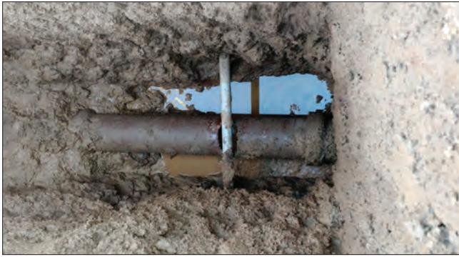
**A fiber optic installation damaged this sewer line. The problem was located during televising the system; the city repaired the problem.**
