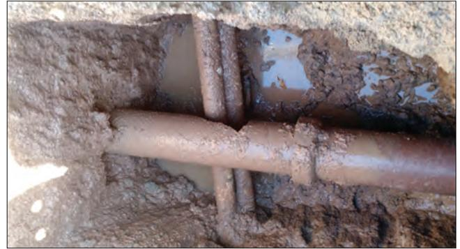
**This photo shows two fiber optic conduits that hit the main; repairs were made by the city.**
