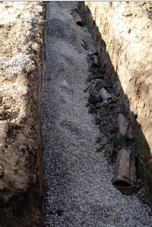
**Photo at top left shows forty feet of main that was replaced; the original pipe failed because it was not bedded. Bedding was added to this section.**
