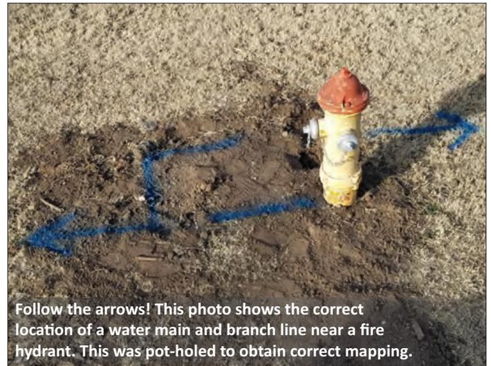
Follow the arrows! This photo shows the correct location of a water main and branch line near a fire hydrant. This was pot-holed to obtain correct mapping.
