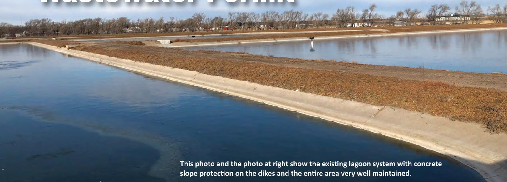
This photo and the photo at right show the existing lagoon system with concrete slope protection on the dikes and the entire area very well maintained.
