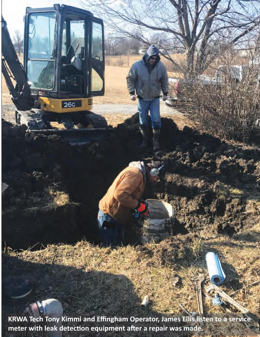
KRWA Tech Tony Kimmi and Effingham Operator, James Ellis listen to a service meter with leak detection equipment after a repair was made.
