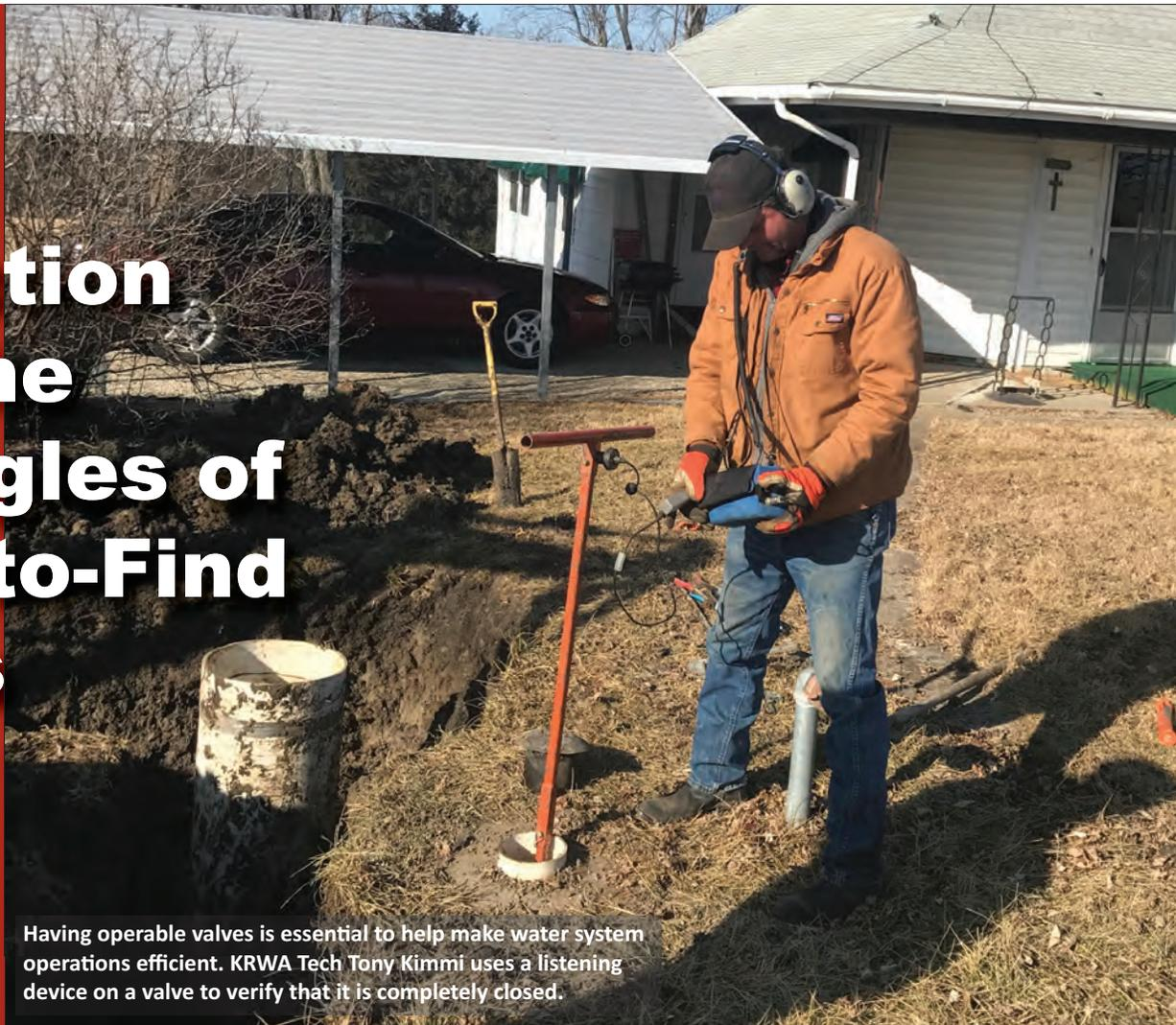
Having operable valves is essential to help make water system operations efficient. KRWA Tech Tony Kimmi uses a listening device on a valve to verify that it is completely closed.
