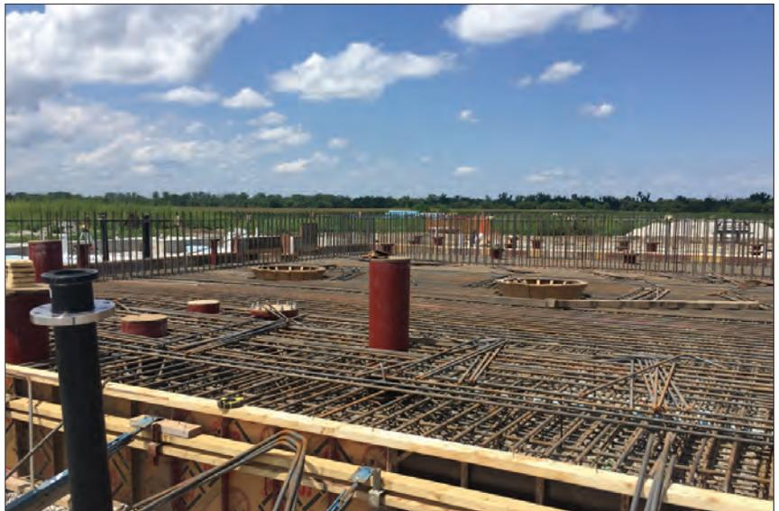
**This photo shows the immense amount of reinforcing bar that was installed in the flooring of the water treatment plant.**
