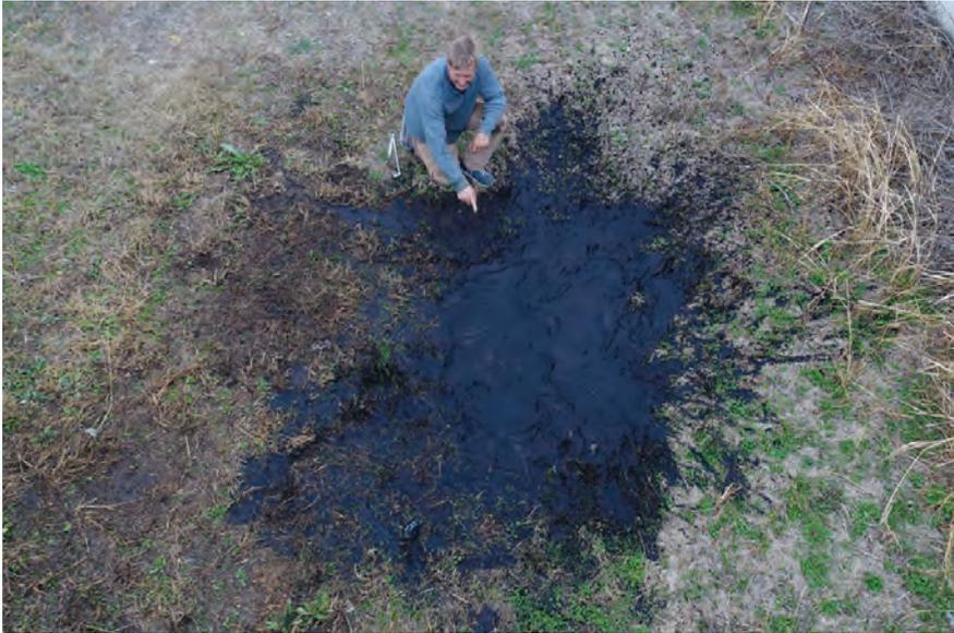
**KRWA Tech Assistant Jon Steele points to the manganese and iron deposits that were removed from the water storage standpipe. The tank had not been cleaned since the system was constructed. In the photo at right, Steele is vacuuming the deposits from the tank.**
