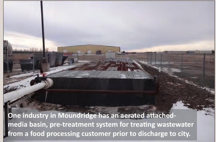
One industry in Moundridge has an aerated attached-media basin, pre-treatment system for treating wastewater from a food processing customer prior to discharge to city.
