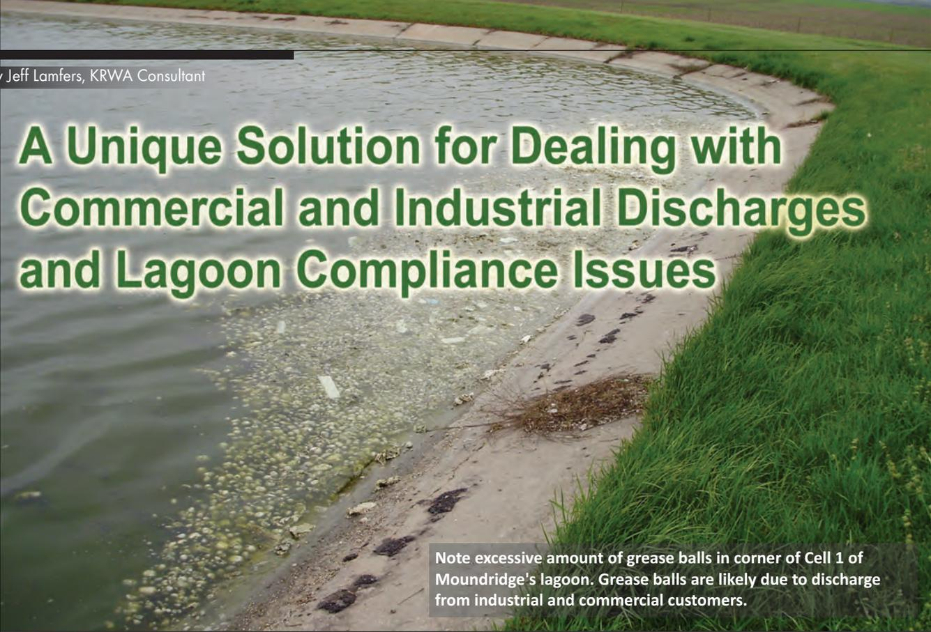
Note excessive amount of grease balls in corner of Cell 1 of Moundridge's lagoon. Grease balls are likely due to discharge from industrial and commercial customers.
