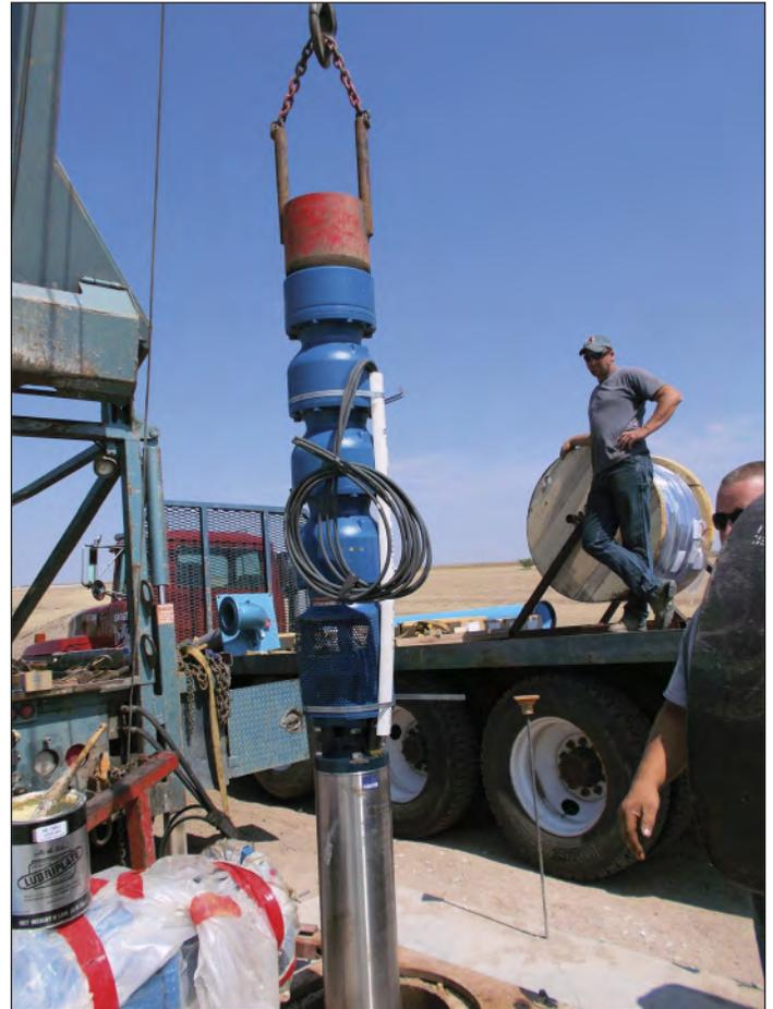
The new submersible well pump with a 125 HP motor, which while capable of delivering 750 gpm, will be set to deliver 550 gpm to the system.
