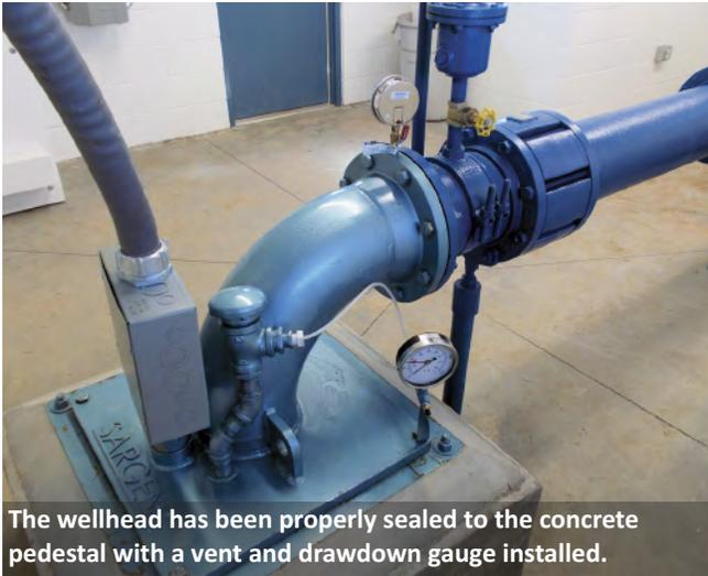
The wellhead has been properly sealed to the concrete pedestal with a vent and drawdown gauge installed.
