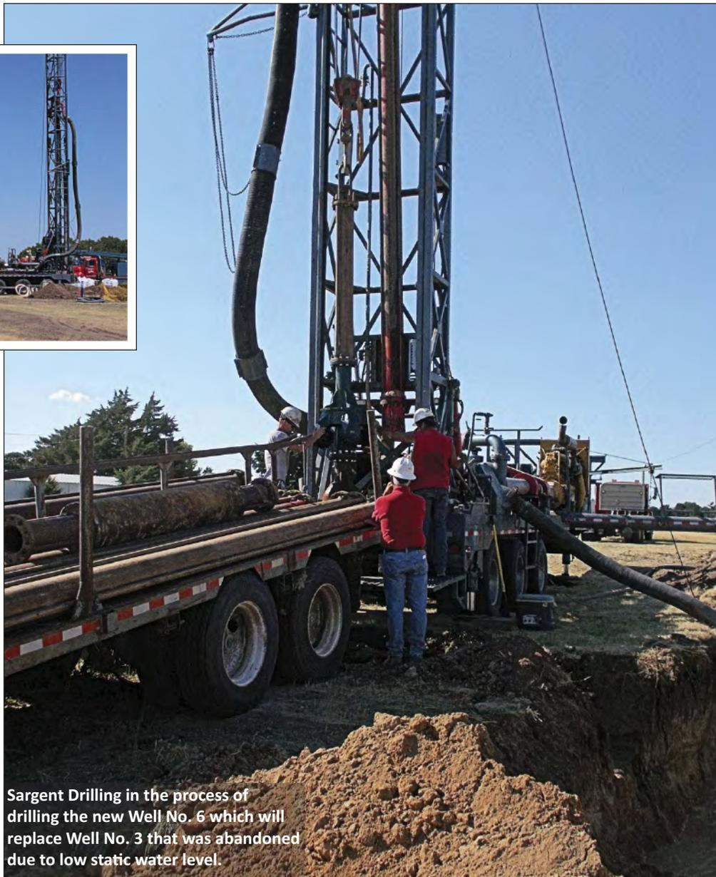
Sargent Drilling in the process of drilling the new Well No. 6 which will replace Well No. 3 that was abandoned due to low static water level.
