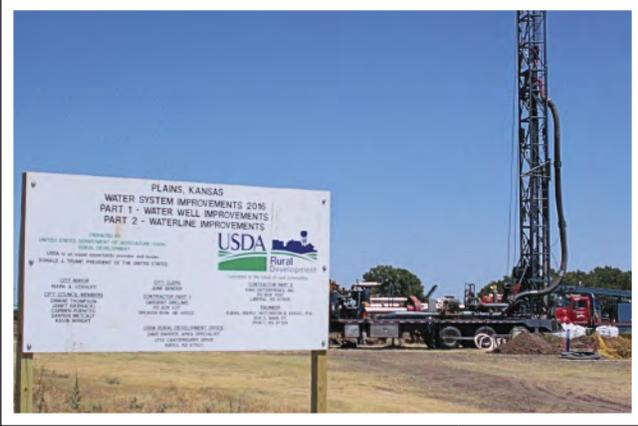
This photo with the USDA Rural Development project sign in the foreground, shows Sargent Drilling in the process of drilling the new Well No. 6 which will replace Well No. 3 that was abandoned due to low static water level.
