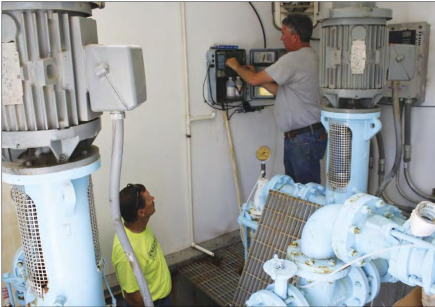
**RWD Operator Roger Engemann works on installing the injector while KRWA Tech Lonnie Boller works on repairing the chlorine analyzer. A new photocell was also installed and the unit was retubed.**
