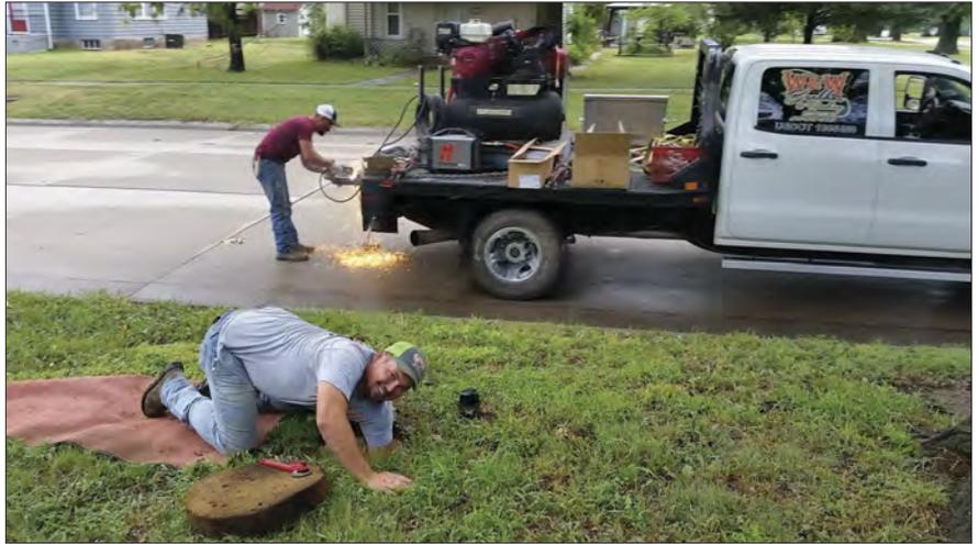
Shane Spencer installs a new meter while Josh Blackburn uses a plasma cutter to cut the hole in the cast iron lid for the antenna. The meter installation was completed by W & W Backhoe and Trenching, Mound Valley, Kansas.
