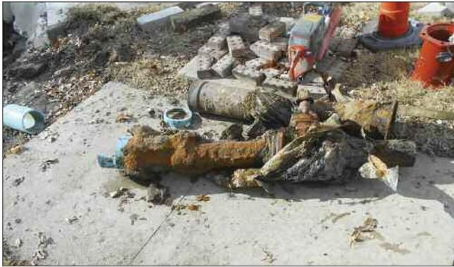
This photo shows a section of old pipe with valve and valve box which was removed.
