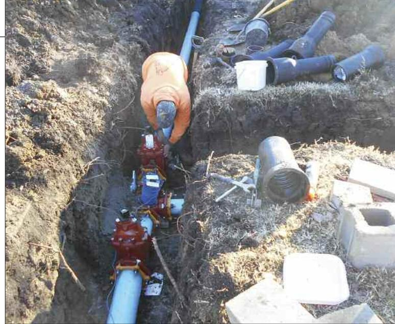
Water pipeline with valves is being installed along with tracer wire. Valve risers are shown in this photo also.
