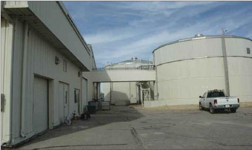
**This photo shows the surface water treatment plant with two covered clarifiers and the building to the left housing filters, chemical room, laboratory, and office. Water from Marion Reservoir is treated by Hillsboro which also sells water to the city of Peabody.**
