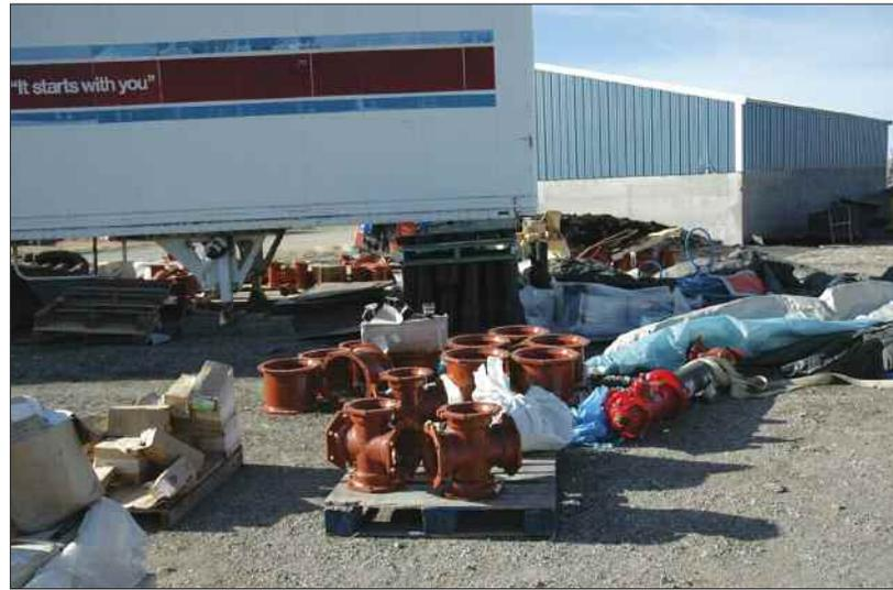
Shown here are fittings and a fire hydrant still to be installed. All fittings used in this project were epoxy-coated to protect against corrosion.
