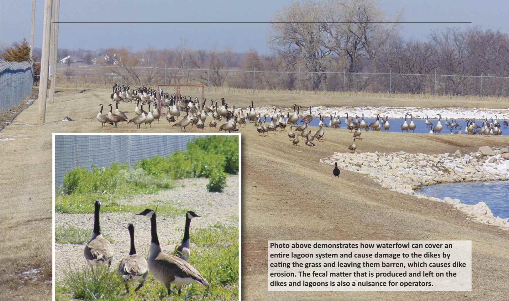
Photo above demonstrates how waterfowl can cover an entire lagoon system and cause damage to the dikes by eating the grass and leaving them barren, which causes dike erosion. The fecal matter that is produced and left on the dikes and lagoons is also a nuisance for operators.
